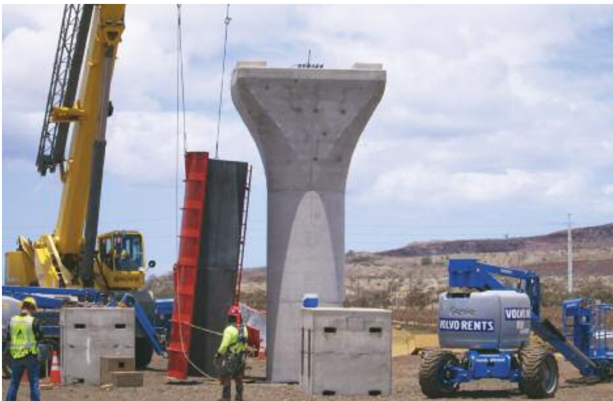
Kiewit Infrastructure West | Photo courtesy Honolulu Authority for Rapid Transportation (HART)
