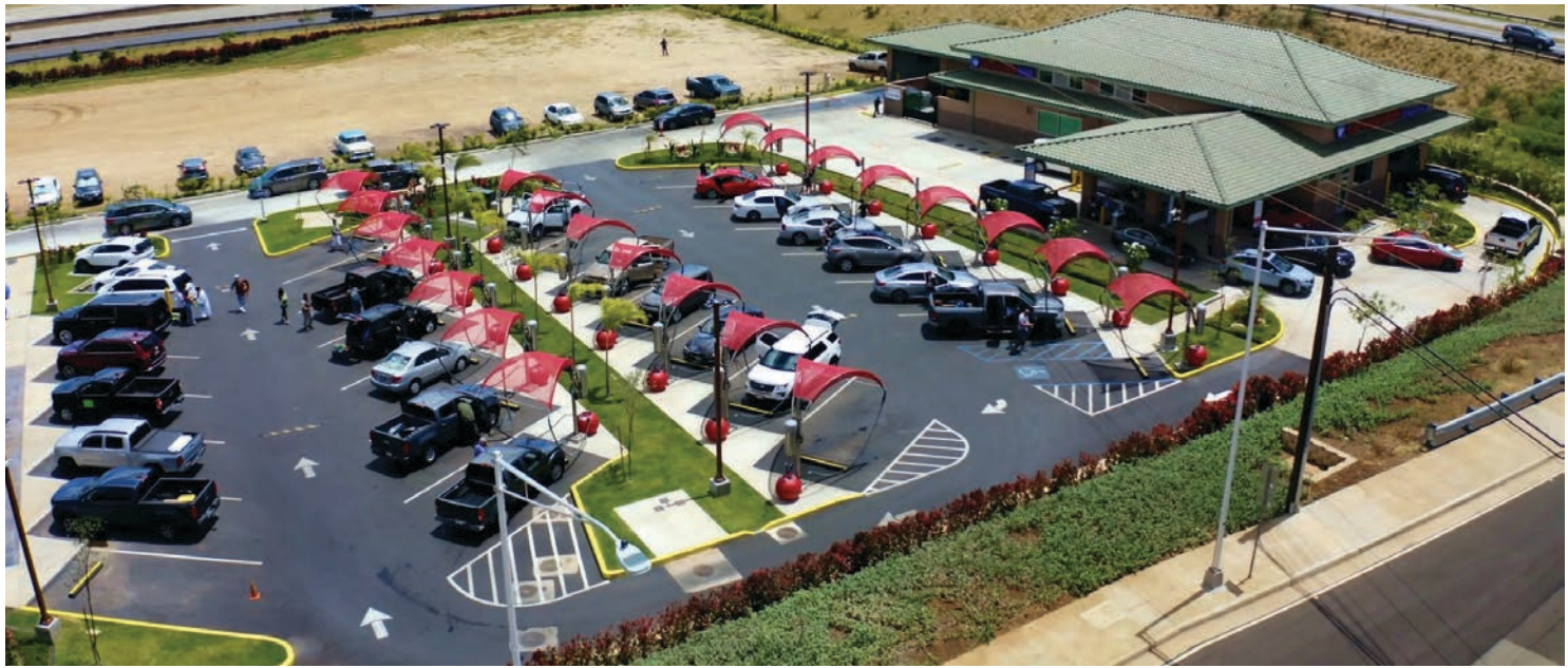
PHOTOS COURTESY OF CARWASH808 EXPRESS
